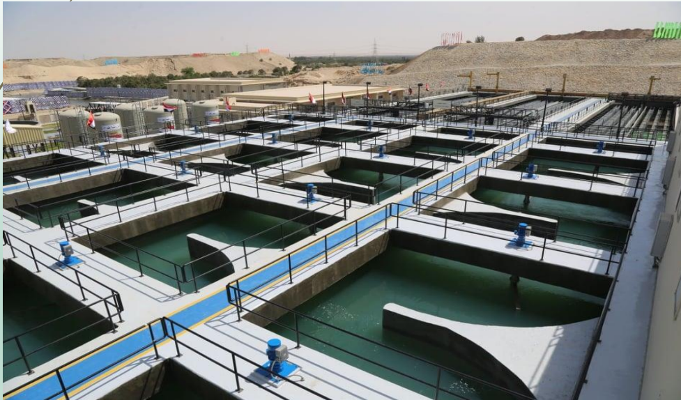
Al Mahsama agricultural drainage treatment, recycling and reuse plant – Ismailia governorate.
